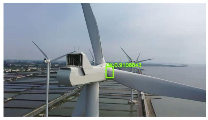
It is possible to use drone photography combined with Solomon Al recognition to detect whether components of wind turbine blades have detached.
